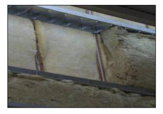
Picture showing the two layers of new insulations (50 + 100 mm), and the steel frame for the panels.
