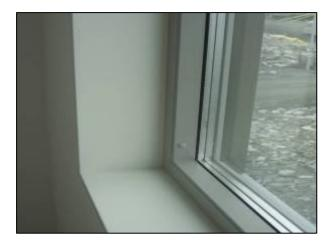
Energy efficient windows with triple glazing. 2 low emission coatings, argon gas, superspacers and wooden frame. This construction gives a U-value of 0.95  $W/m^2K$ .
