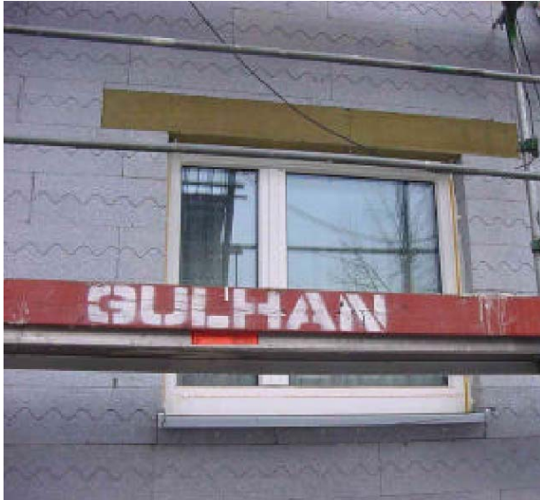
Fig. 1: Insulation of window lintels with mineral wool
