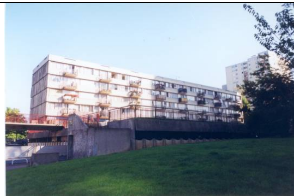
Building before renovation (2000)
