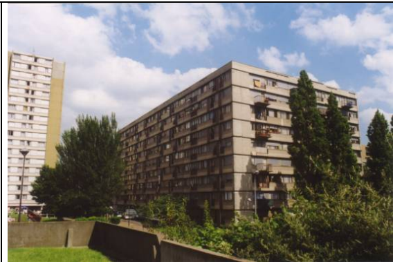
Neighbouring buildings (east and south)
