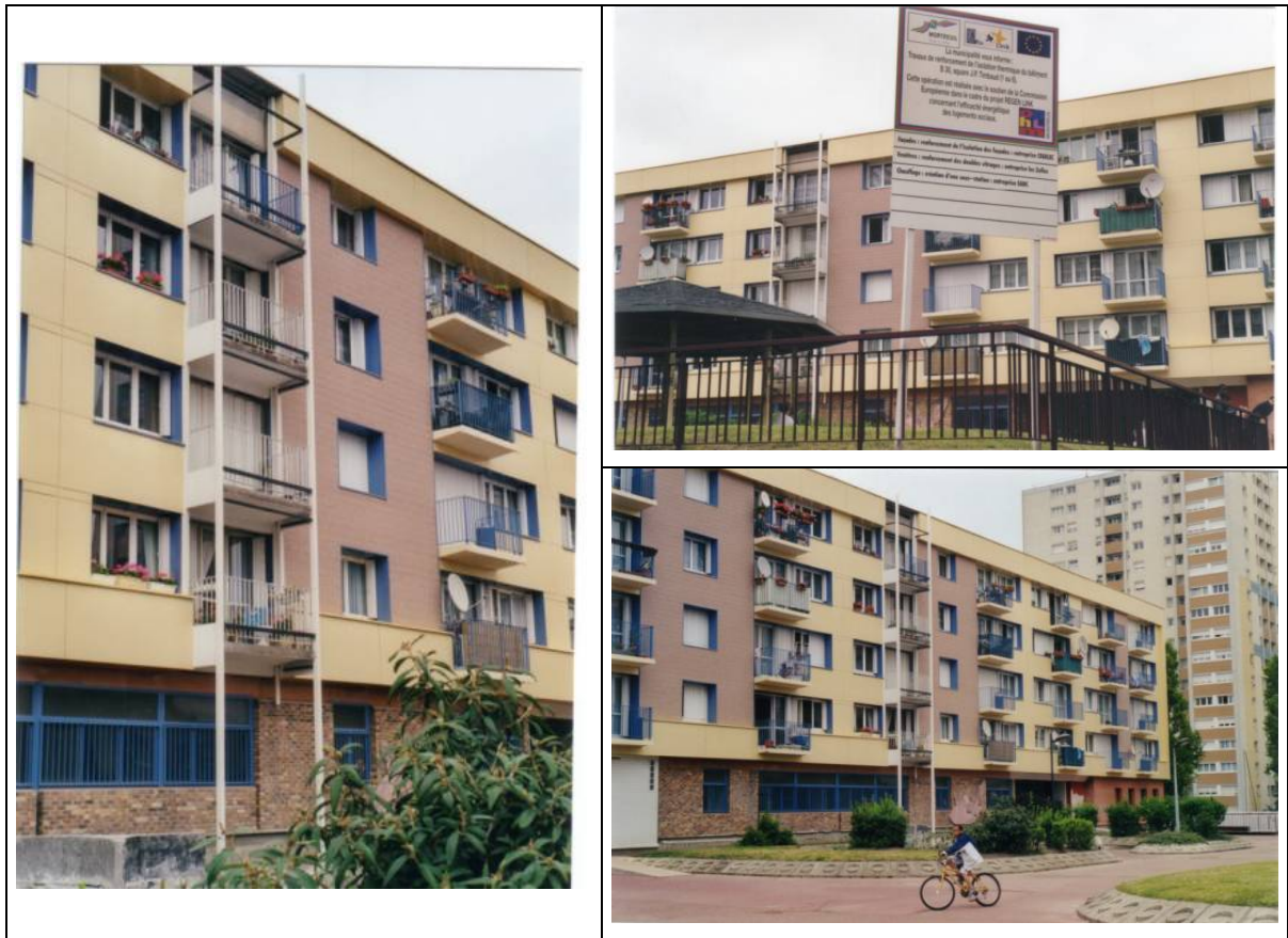
The renovation of the building has been completed with the installation of the glazed balconies in autumn 2002 (see the next photographs) by the company TRADIRENOV.
