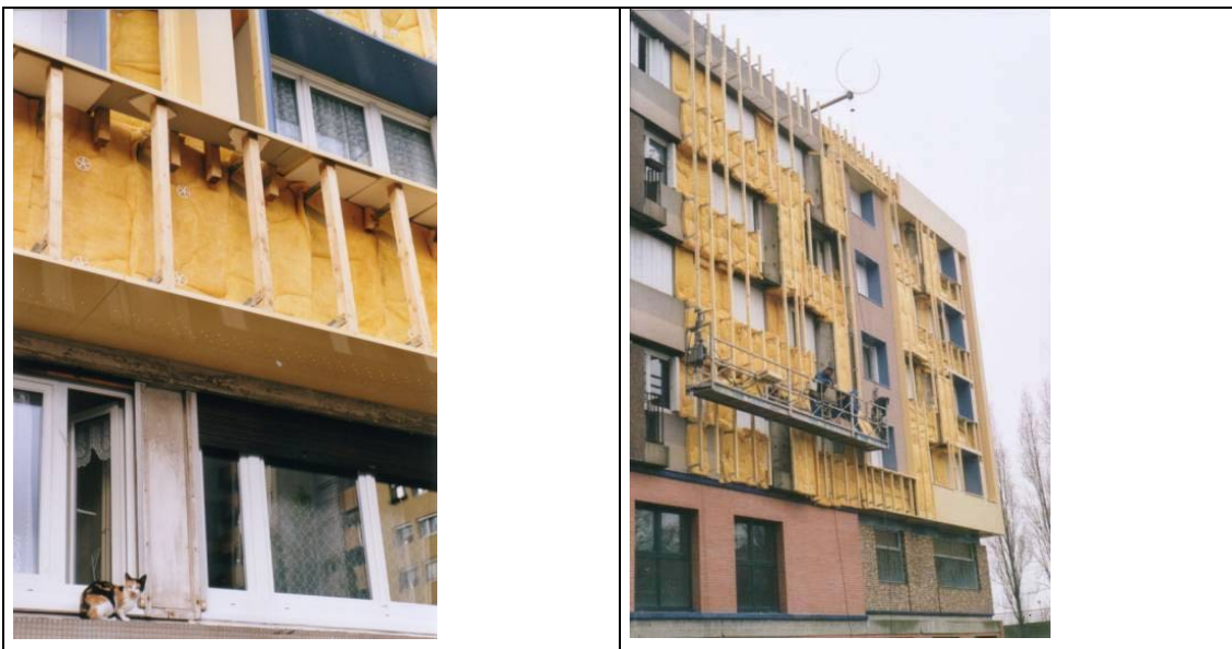
View of the building site, implementing the external insulation
