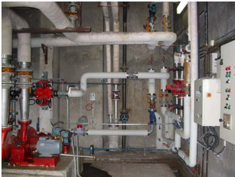
New heating loop (district heating connection)
