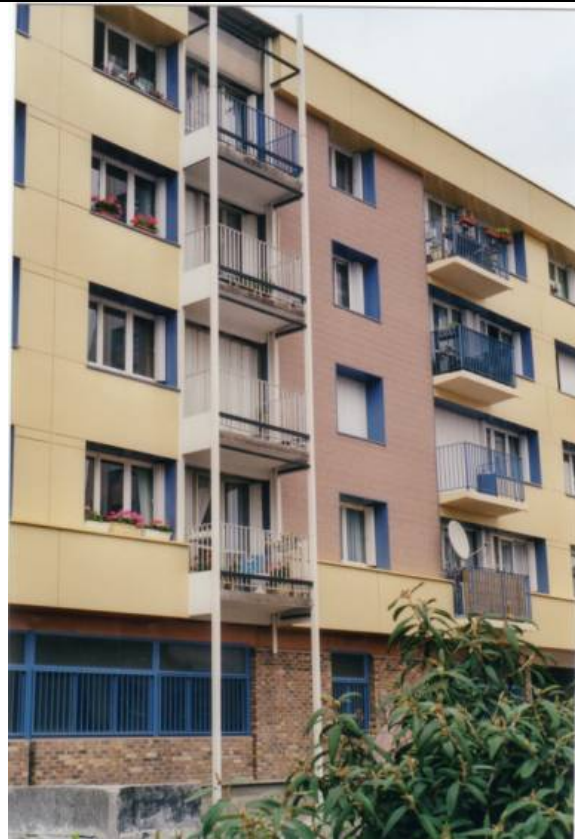
Renovation of the glazed balconies (July 2002)
