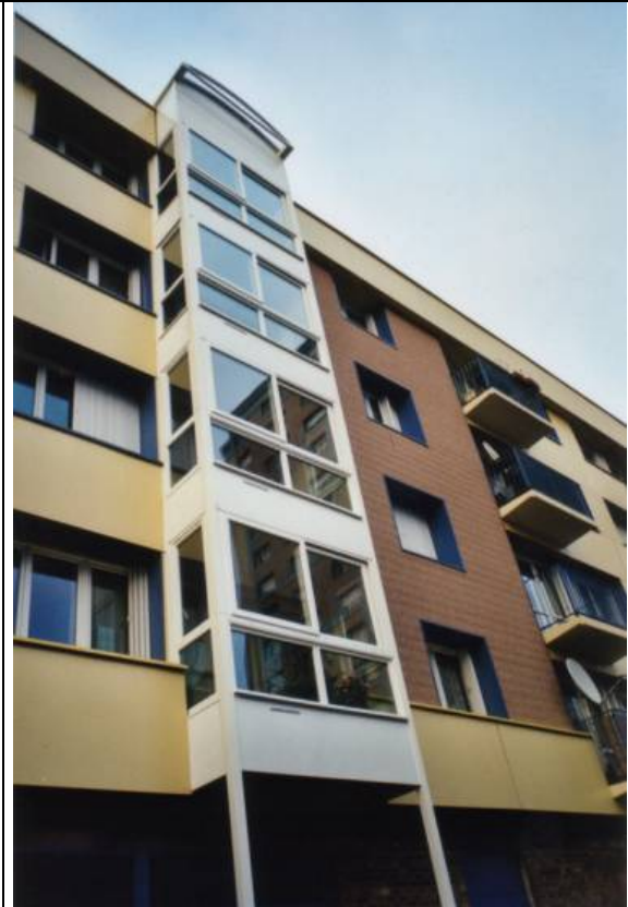
Renovation of the glazed balconies (December 2002)
