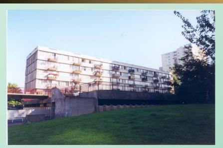
Construction: 1969, not insulated, single glazing heating load: 150 kWh/m²/a (2,700 degree days base 18)
