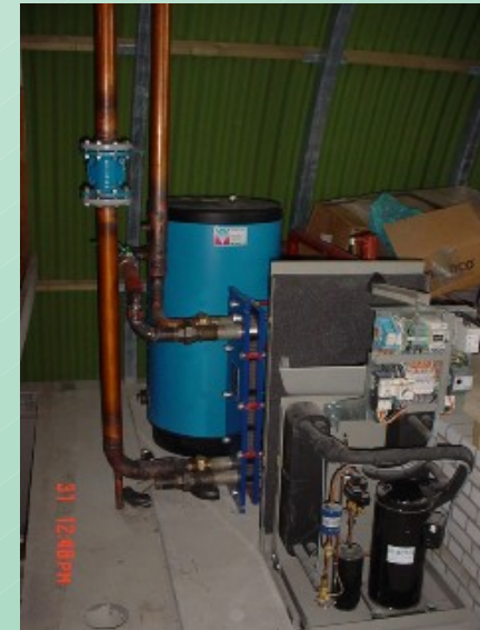
Heat exchanger on roof (left) and heat pump (right)
