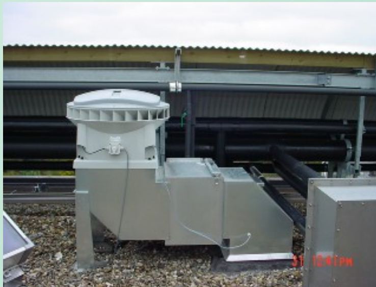
Heat exchanger on roof (left) and heat pump (right)
