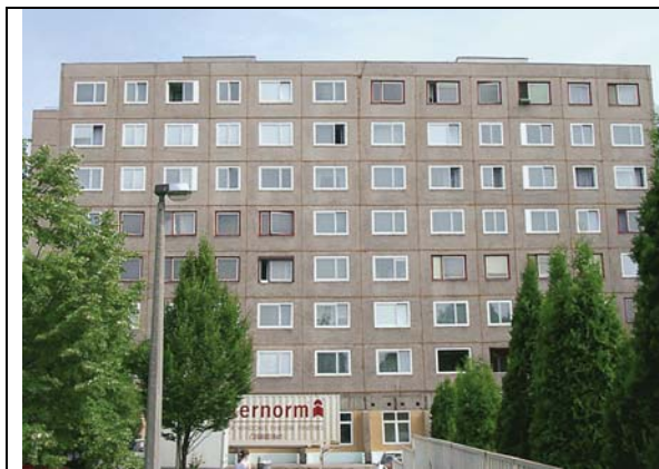
Figure 1: The Solanova building before renovation
