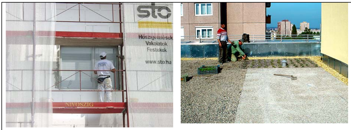
Figure 3: The facades were covered with 16 cm polistyren thermal insulation
