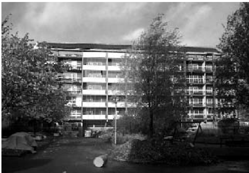
Fig. 7 High-rise building with roof-integrated collectors and glazed balconies under construction.
