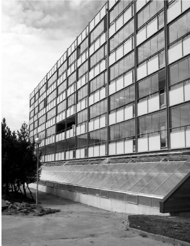
Fig. 6 South facing façade with glazed balconies and greenhouse. Photo: C. Nordström.
