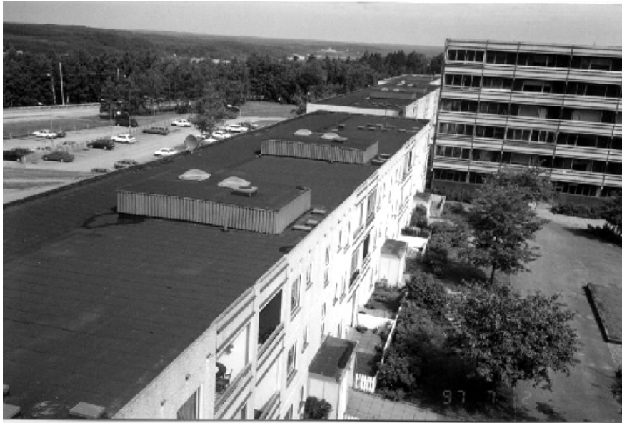
Fig. 2 View from one high-rise building over the yard to northeast. Left: Roof tops with ventilation systems on a low-rise building. Right: High-rise building with balconies facing south.
