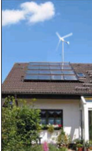
On site renewables with wind energy and photo voltaic solar energy
