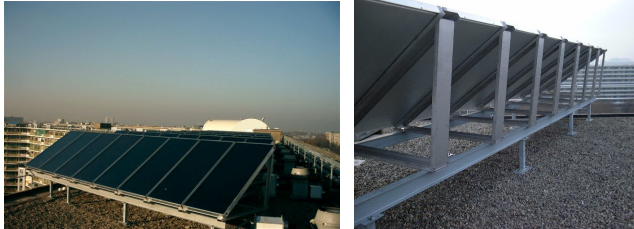
Start of construction 720 m2 collector (left) and framework (right)
