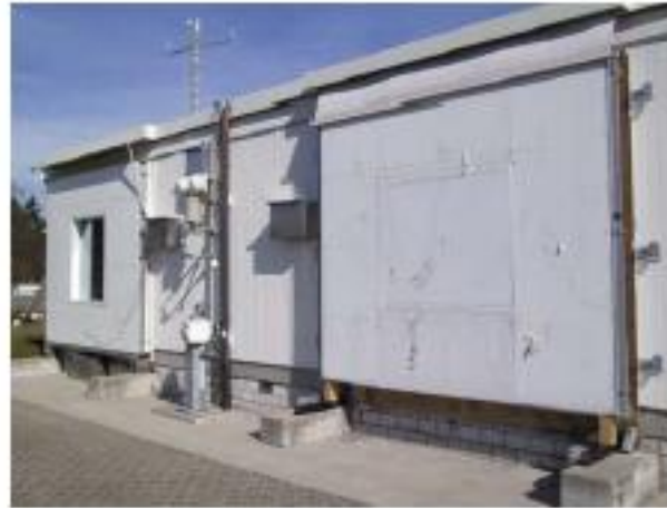
Figure 1a Outdoor test facility with removable façade element.
