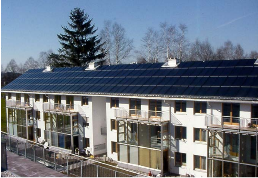
Roof-intergrated solar collectors on multifamily building in Austria Photo: SOLID / Austria Solar
