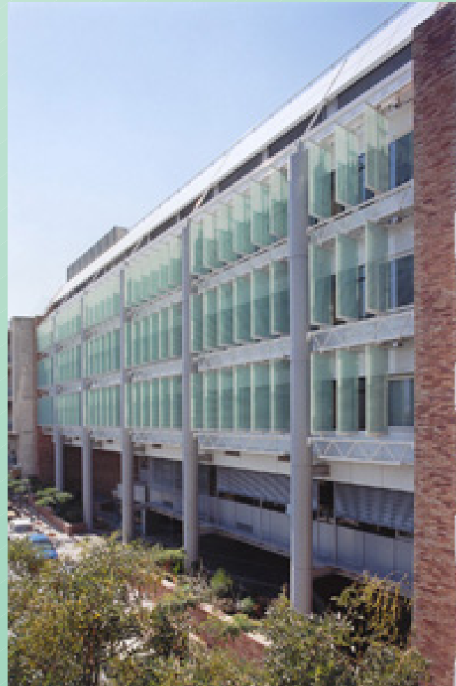
Vertical shading east / west facades Arch. A. TOMBAZIS
