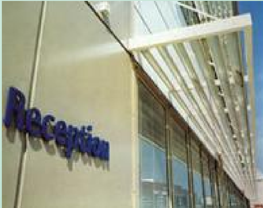
Horizontal shading south facades Zephyr system
